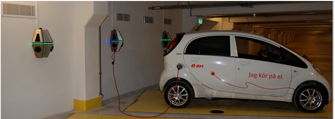
Figure 4 Example of wall mounted installation
