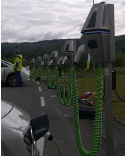
Figure 2 Example of pole mount installation
